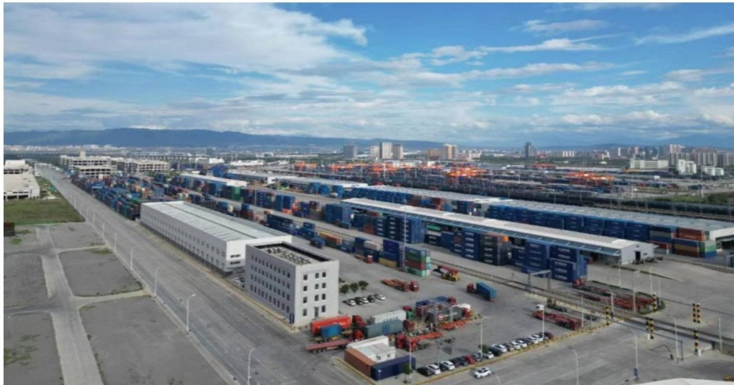
仓库外部区域鸟瞰图 | Aerial view of the warehouse exterior area
